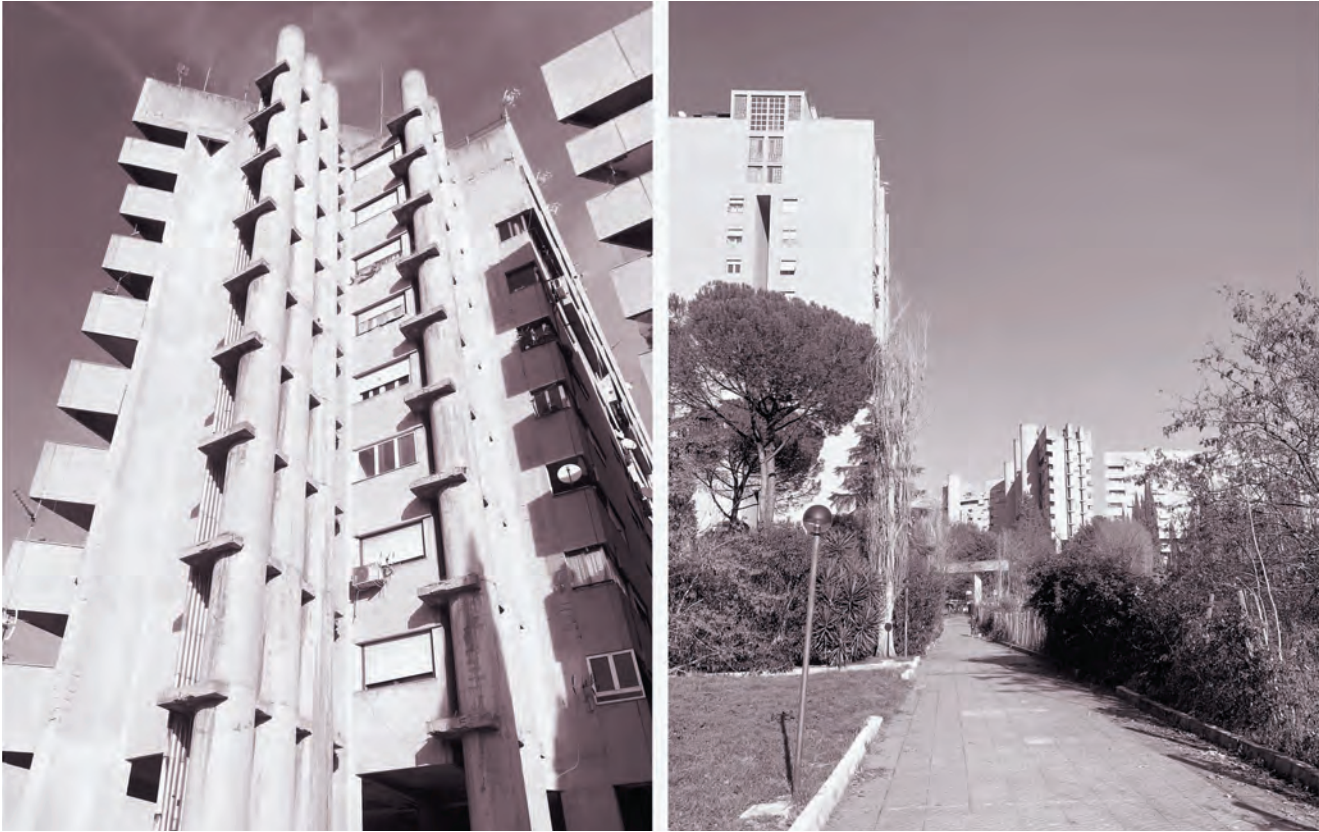
Fig. 2: External views of the Vigne Nuove complex (south-east side)
